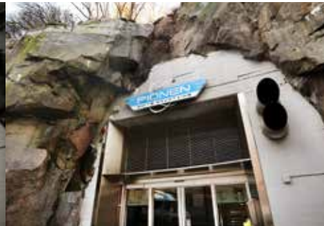
2014: Today the surplus heat is recovered and sold to Stockholm's district heating network.
