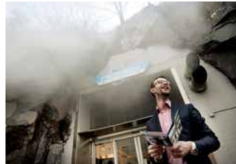
2007: When Bahnhof opened the data centre Pionen the excess heat was released as a plume of steam straight into the street.
